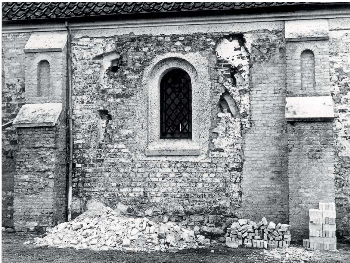
Fig. 21. Sydsiden af skibets østfag under renovering. Øst for 1878-vinduet ses den falsede arkadebue under et blændet, gotisk vindue; vest for vinduet ses rest af 1823-vindue. Foto i NM, 1961. – The south side of the east bay of the nave during renovation. East of the 1878 window one can see the chamfered arcade arch beneath a filled Gothic window recess; west of the window one sees the remains of the 1823 window.
